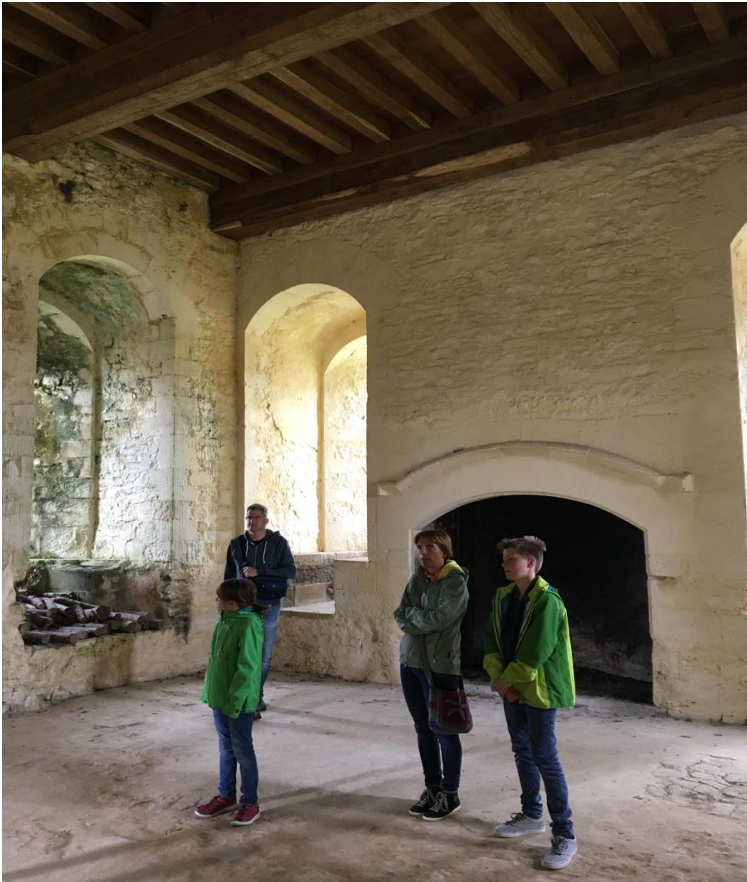
The Keep – interior showing thickness of walls
